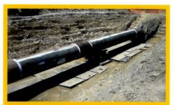
If the Integrity Dig inspection determines a repair is required, the pipe section will be replaced or a pipe sleeve will be welded over the identified portion of the pipe to restore its integrity.
